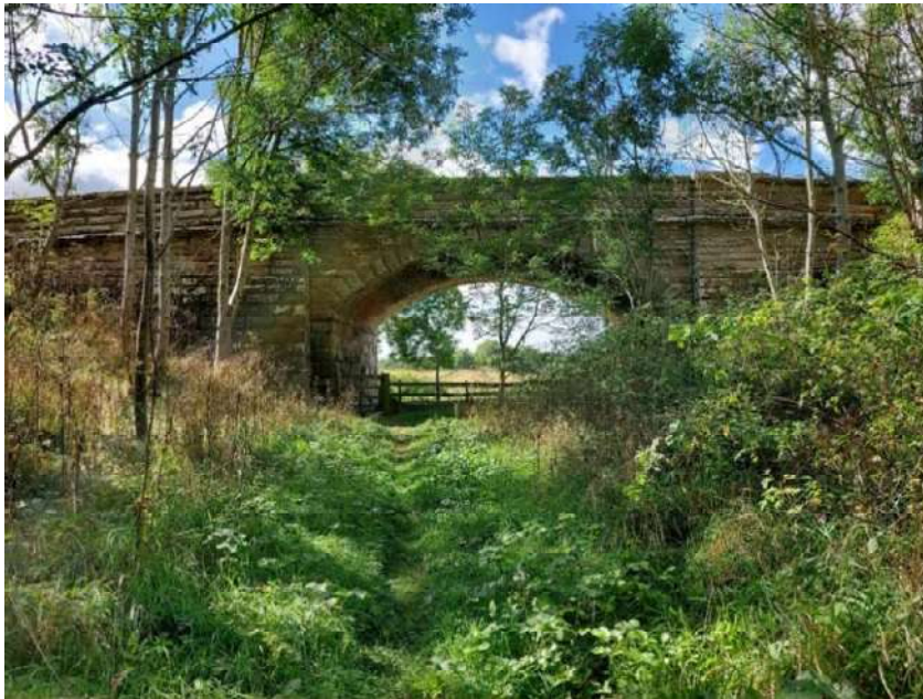
Road bridge over the Railway
